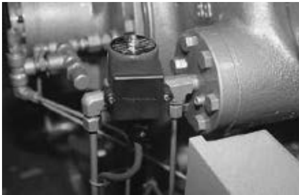
Unloader solenoid valve
